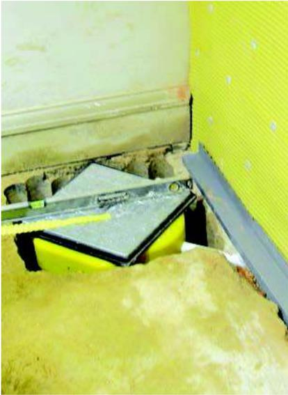
penetrate the basement walls and then fall behind the membrane into a drainage channel. Other than at the baseline, the membrane does not need to be perfectly jointed or sealed to work, because the water penetrating the walls will depressurise when it enters the air gap due to the lower pressure. Unfortunately, this is conducive to enhancing the draw of radon towards the basement.
